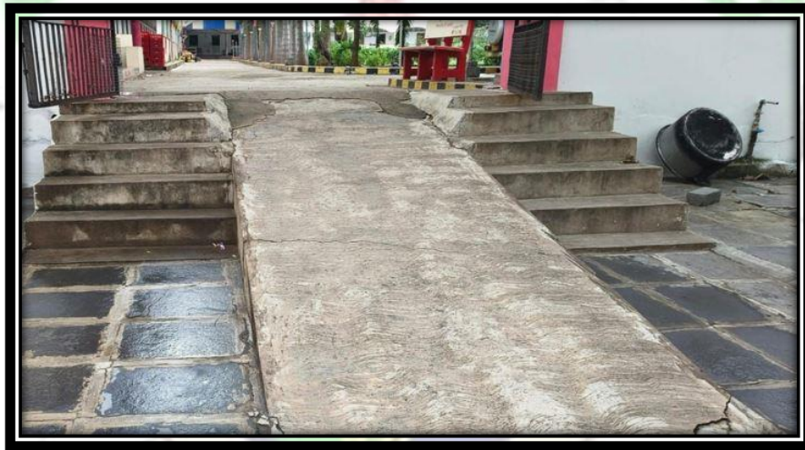
Figure: Ramp for Physically Disabled Person
